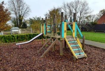
**Finding:** The raised timber edging forms a hard object within the falling space of the equipment and there is also insufficient surfacing provided in contravention of BS EN 1176 Part 1
