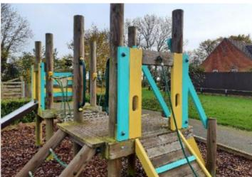
**Finding:** The unit is easily accessible and has an opening in **Action:** Monitor - No remedial work recommended the barrier to steep play elements in excess of 500mm in contravention of BS EN 1176 Part 1
