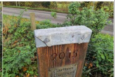
**Finding:** Lead flashing has been used to form a cap on the **Action:** Refer to the supplier for a toxicology assessment top of the sign
