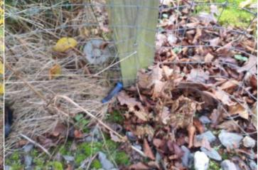
**Finding:** There are areas or parts of the timber posts on the **Action:** Replace all affected timbers structure that have rotted
