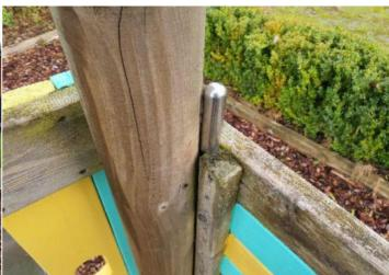
Finding: There is/are finger entrapment/s in the barrier and Action: Monitor - No remedial work recommended the item fails to meet the requirements of BS EN 1176 Part 1
