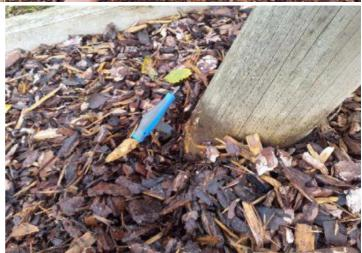
**Finding:** There are areas or parts of the timber support on the structure that have rotted
