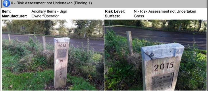
**Finding:** Lead flashing has been used to form a cap on the **Action:** Refer to the supplier for a toxicology assessment top of the sign
