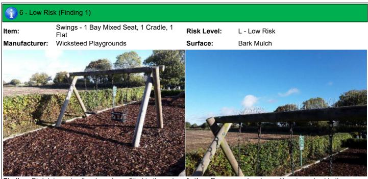
**Finding:** Bird deterrent spikes have been fitted to the swing **Action:** Remove and replace with upturned cable ties and present hazards
