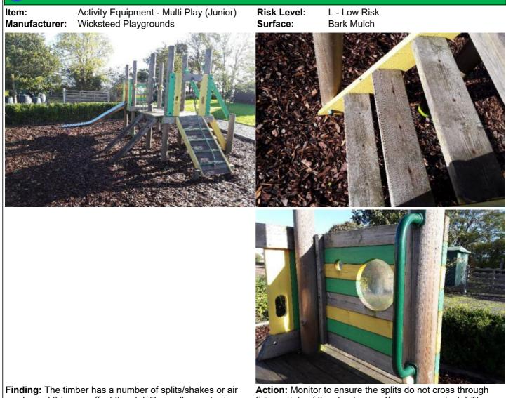
**Finding:** The timber has a number of splits/shakes or air cracks and this may affect the stability or allow water ingress fixing points of the structure and/or cause any instability which will accelerate the rotting process
