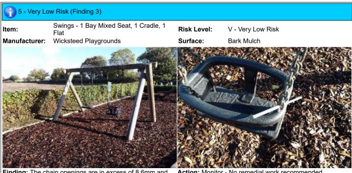
**Finding:** The chain openings are in excess of 8.6mm and do not meet the recommendations of BS EN 1176 Part 1
