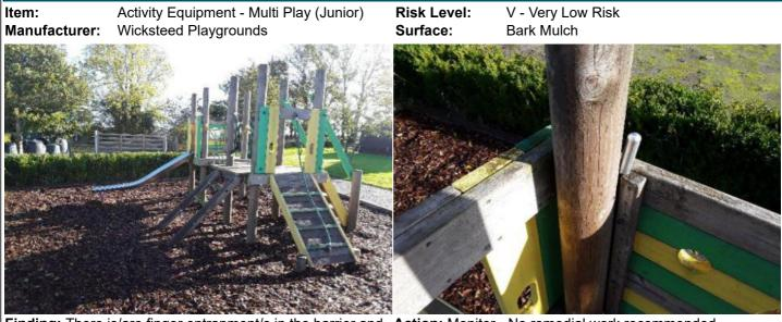
**Finding:** There is/are finger entrapment/s in the barrier and **Action:** Monitor - No remedial work recommended the item fails to meet the requirements of BS EN 1176 Part 1 4.2.7.6 Entrapment of fingers
